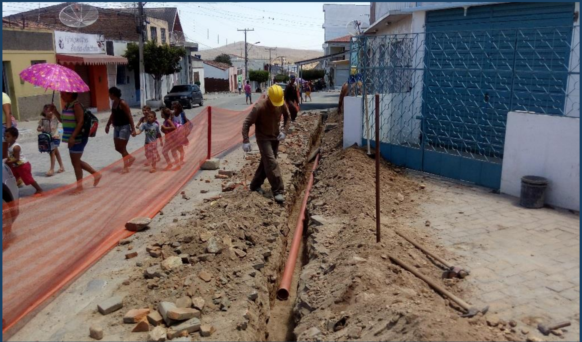
Sidewalk Branch construction – Tacaimbó - Brazil
