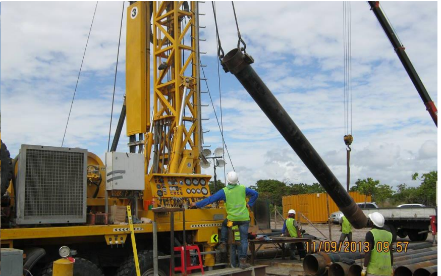
Reverse Circulation Drilling to 600m in 7 Exploration Boreholes
