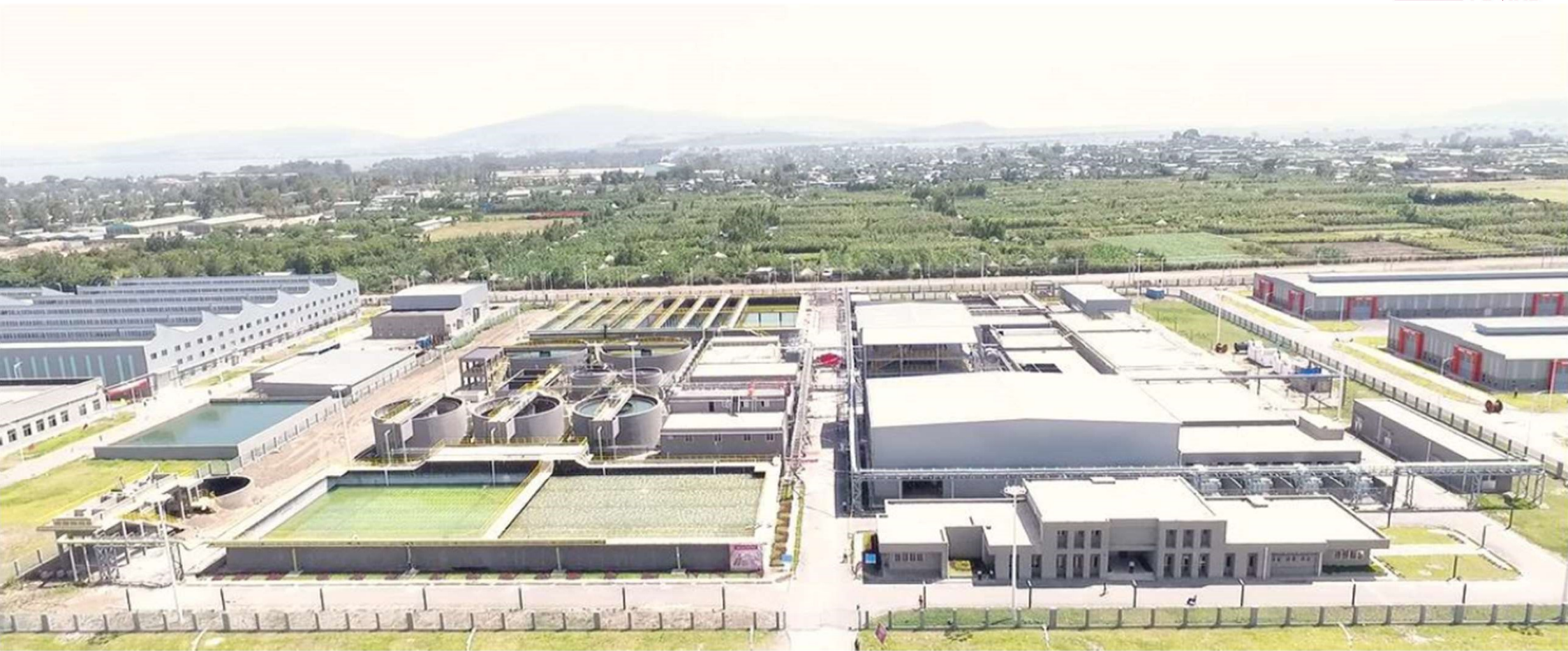
11 MLD Zero Liquid Discharge Plant at Hawassa Industrial Park, Ethiopia
