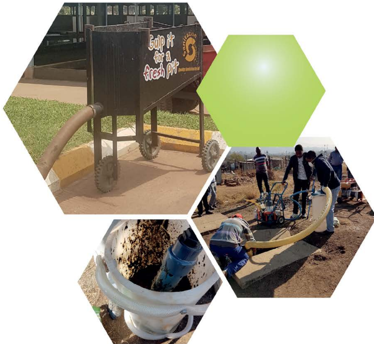
▲ Figure 4 : Semi-mechanized pit emptying
