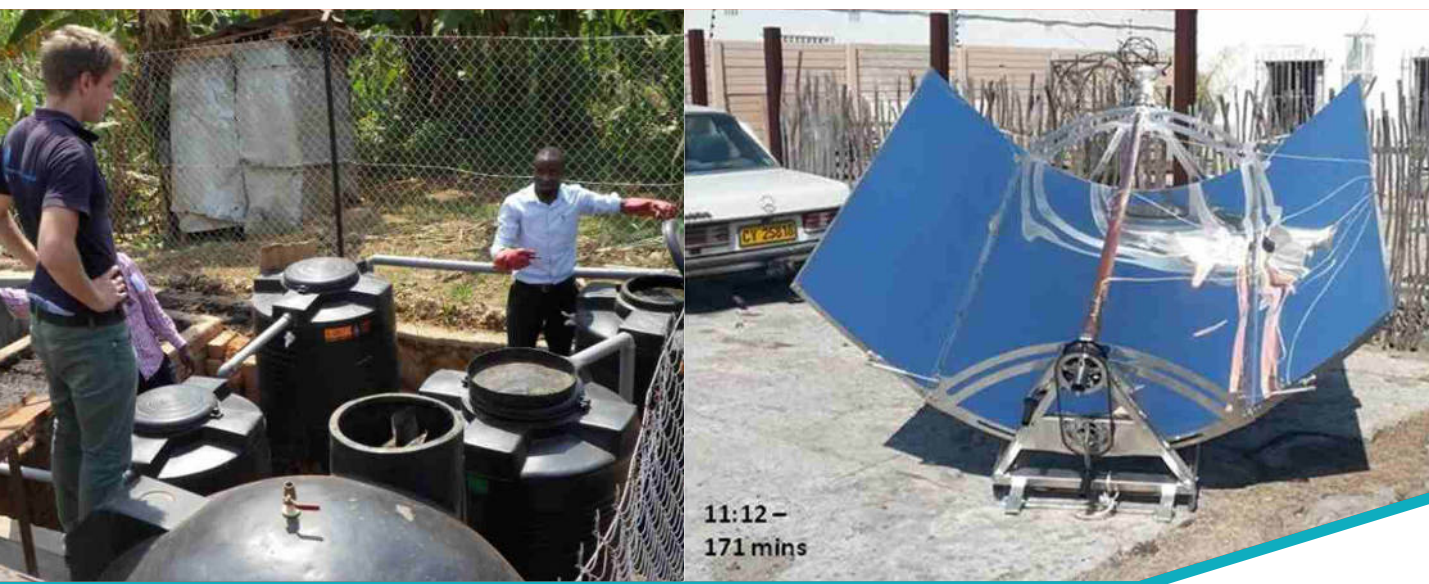
Decentralised anaerobic plant for pit emptiers to reduce transportation costs (Photo: Water for People, Uganda)
