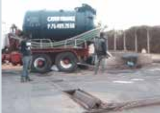
Damaged liquid recovering drain
