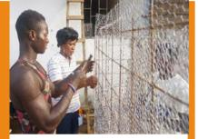
Fabricating the metal cage, that is, the structural support for the tank. Metal cages can be fabricated off-site for mass production and cost-saving purposes.
