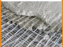
Wire mesh and mortar make an exceptionally strong and waterproof structure. Thinner and lighter than typical concrete construction.
